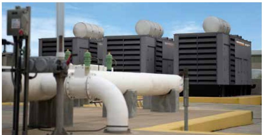
*Generac Industrial Power 3 x 1000 kW Modular Power System (MPS)*
