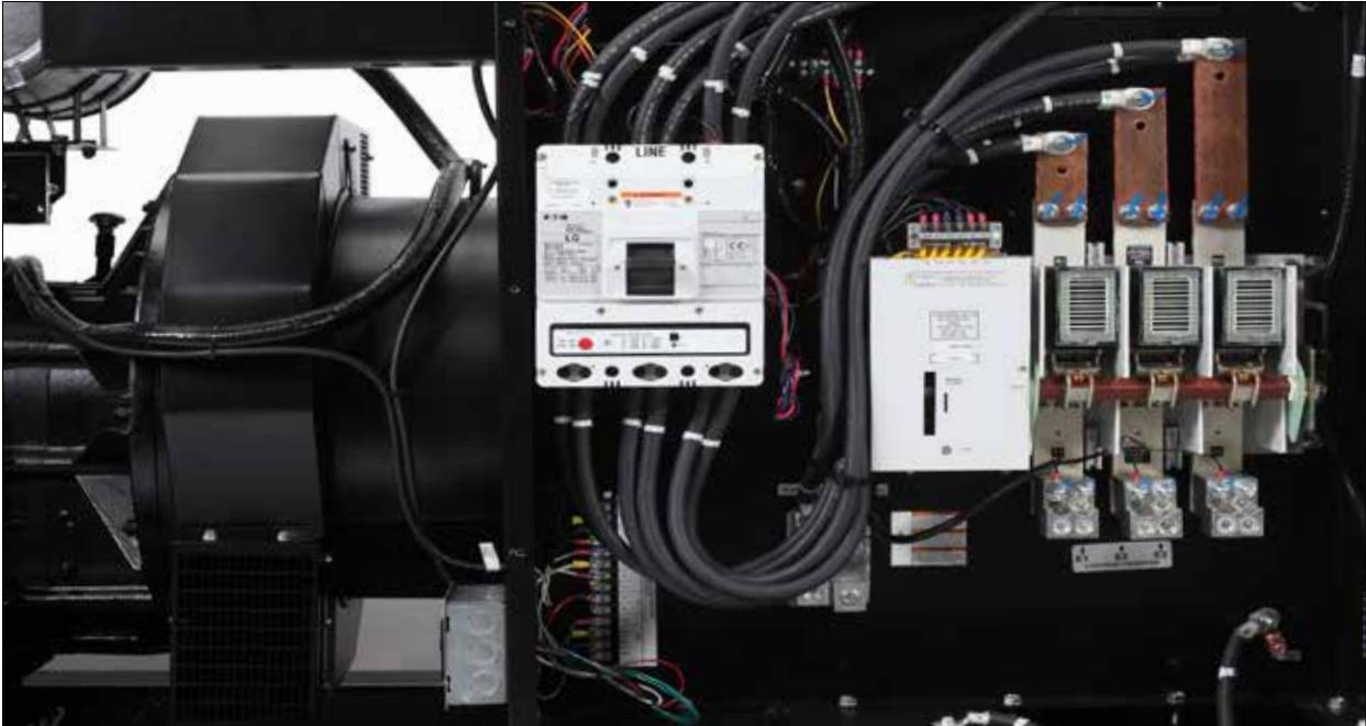
*Paralleling Switching Device located on the generator.*
